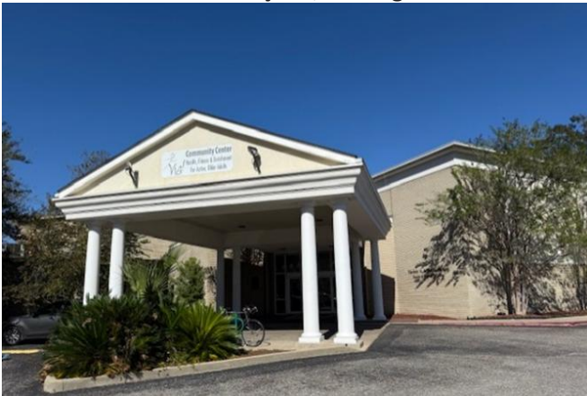
3. Primary entrance from south parking lot, looking N
