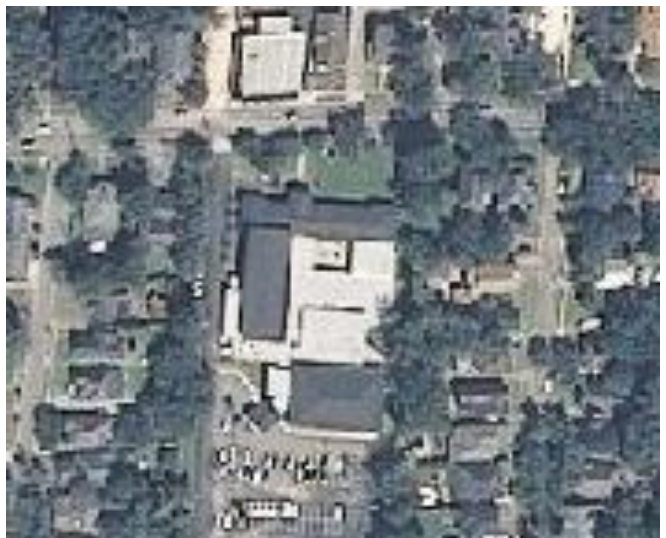
6. Aerial view in 2009, after c. 1990 additions
