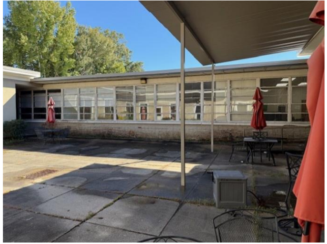
8. View of subject window, looking SE
