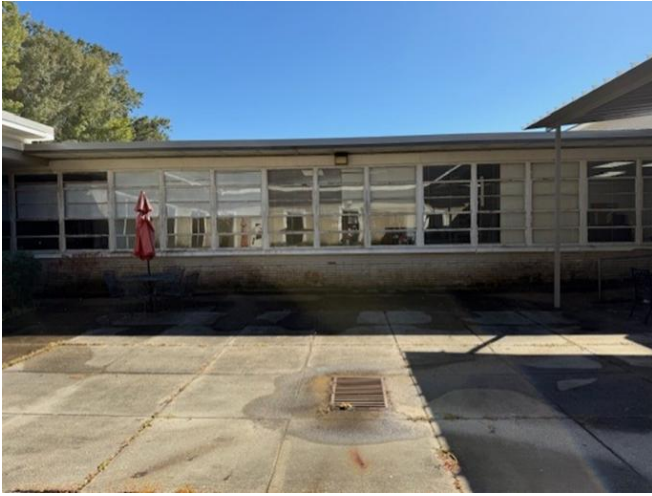
7. View of subject windows, looking S
