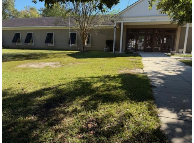
2. View of north façade, looking S
