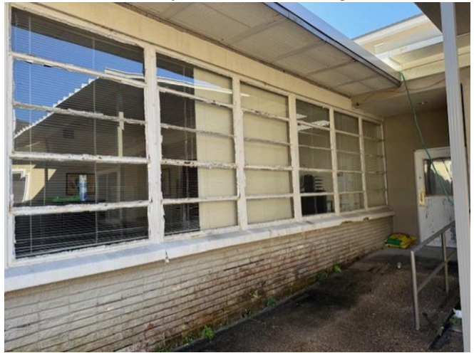
10. View of subject window, looking SW
