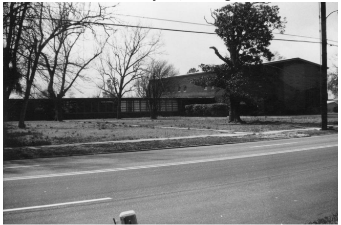
4. View of north façade in 1984 with subject windows visible
