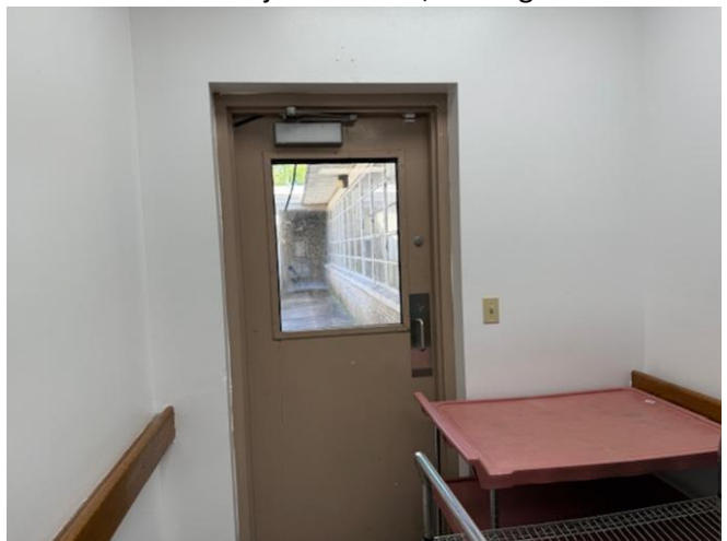
12. Door to interior courtyard where subject windows are located
