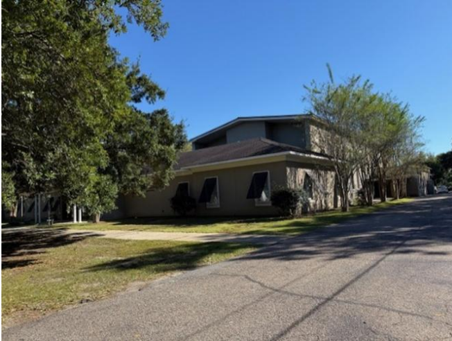
1. View of north façade, looking SE
