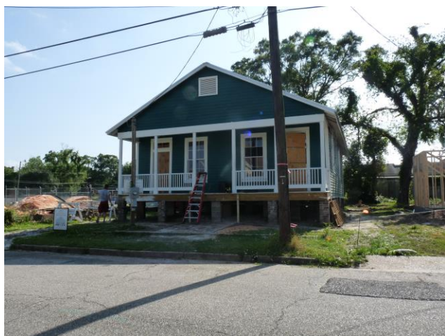
5. View of historic home at 259 N. Dearborn, undergoing rehabilitation
