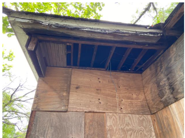
6. Detail of rear elevation
