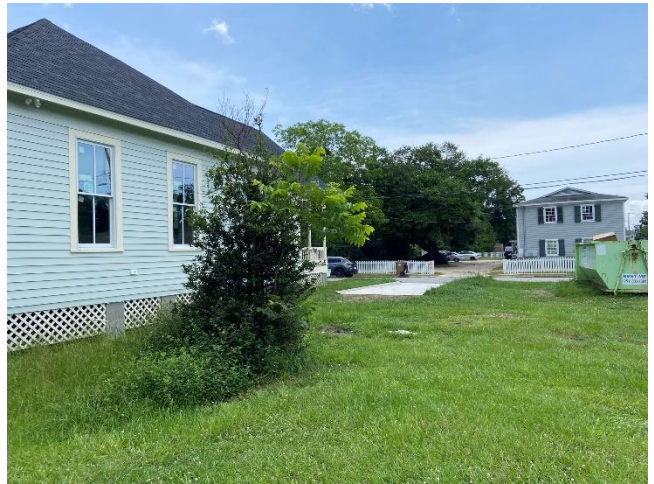
4. Driveway and south side yard, looking west
