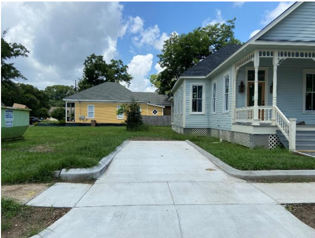
3. Driveway and south side yard, looking west
