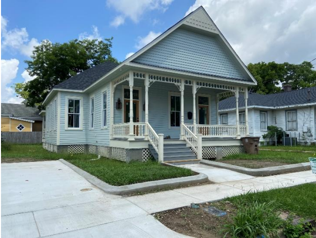
1. East (primary) façade, looking northwest
