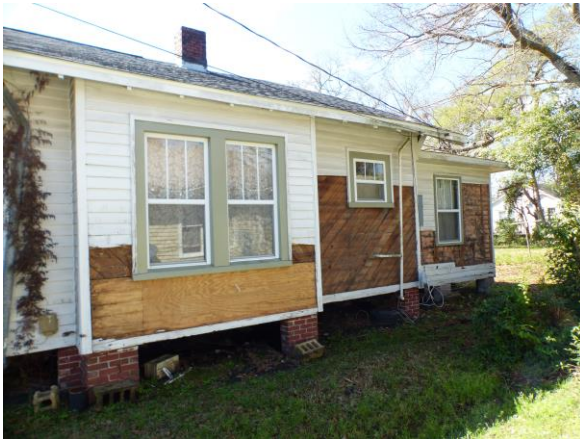
3. View of north elevation
