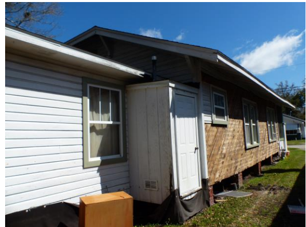
4. View of south elevation
