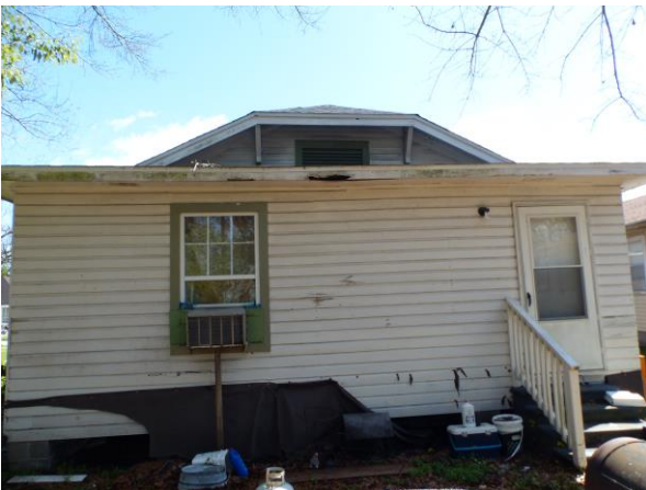
5. View of rear elevation
