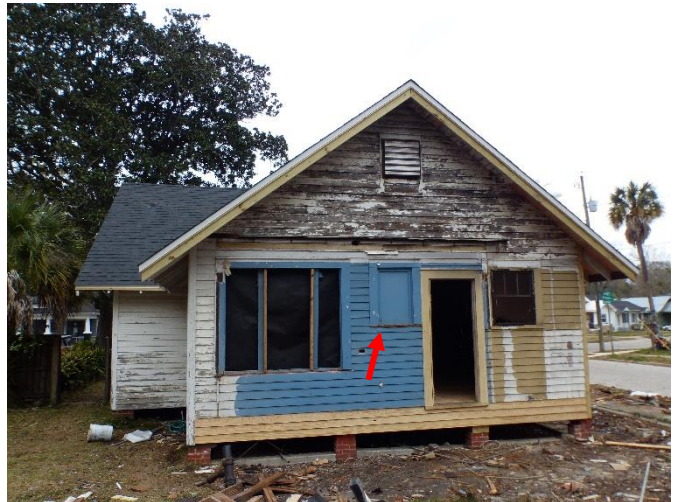
4. East (rear) elevation, looking west. Arrow indicates window proposed for infill.
