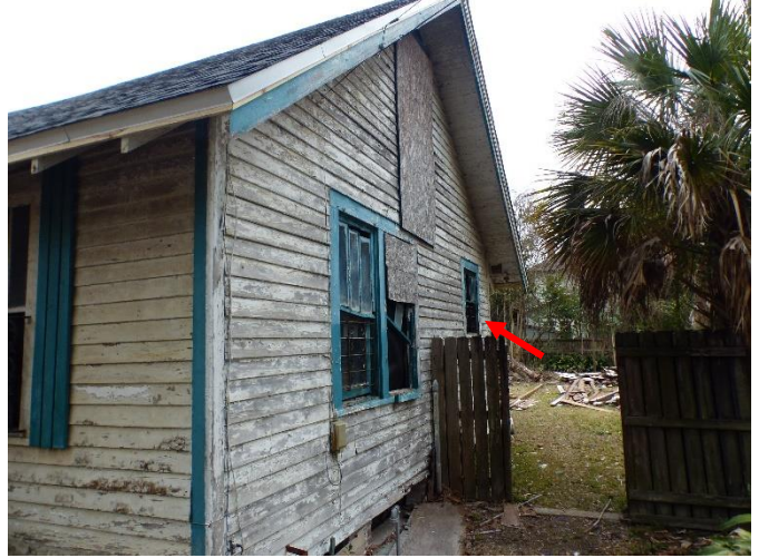
2. South elevation, looking northeast. Arrow indicates window proposed for infill.
