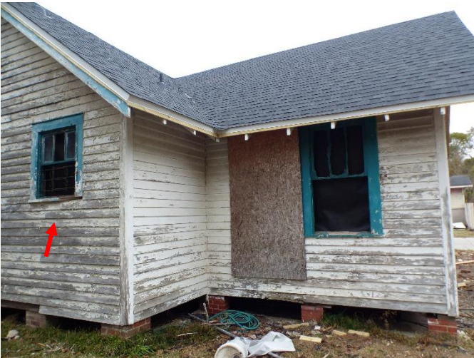
3. South elevation, looking northwest. Arrow indicates window proposed for infill.
