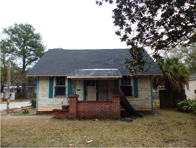
1. West (front) façade, looking east
