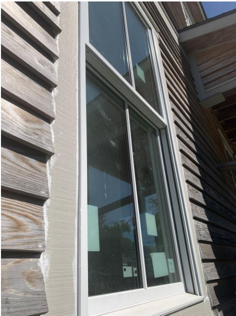
9. Detail: replacement window on south elevation of subject property (October 2023)
