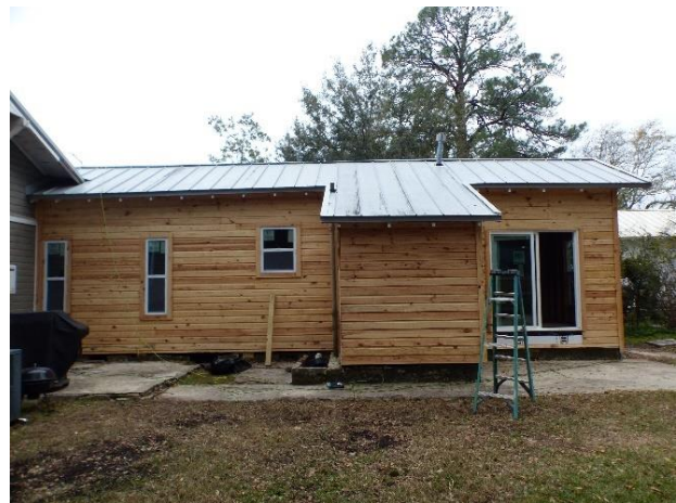
6. View of north elevation
