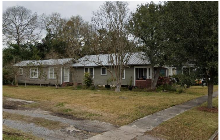
2. South elevation prior to alteration
