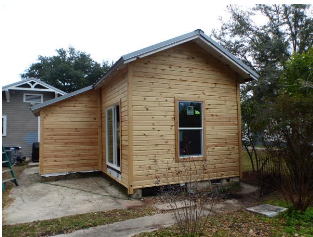
5. View of west elevation of addition
