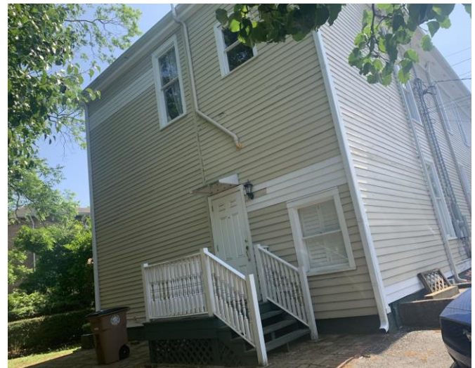
4. View of rear elevation.
