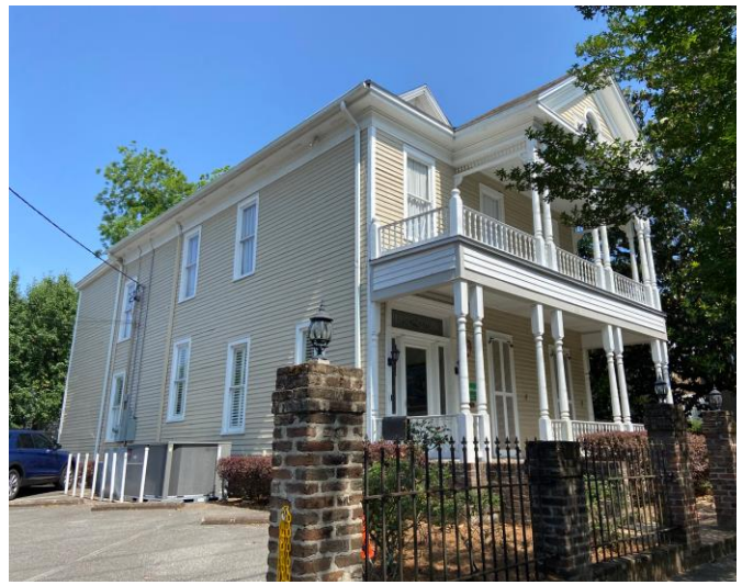
2. View of west façade (right) and north elevation (left)
