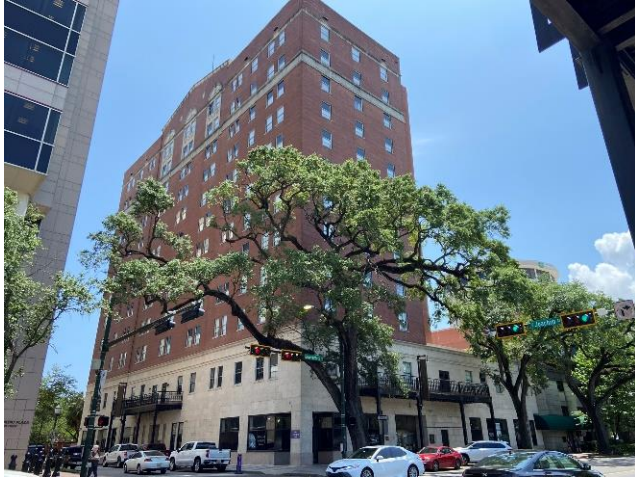
1. North and east elevations, looking southwest
