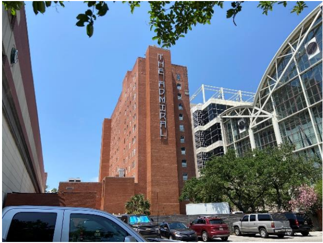
3. South and west elevations, looking northeast
