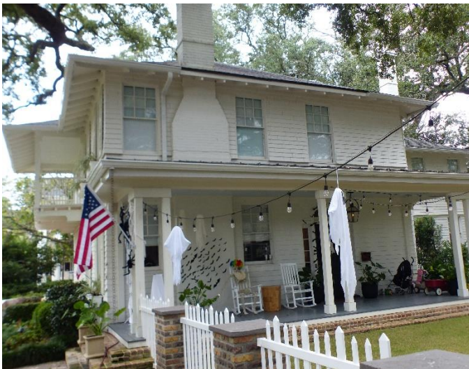
3. Southern end of east elevation
