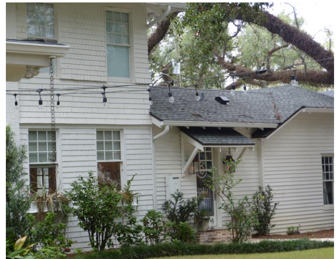
4. East elevation where proposed addition would be placed
