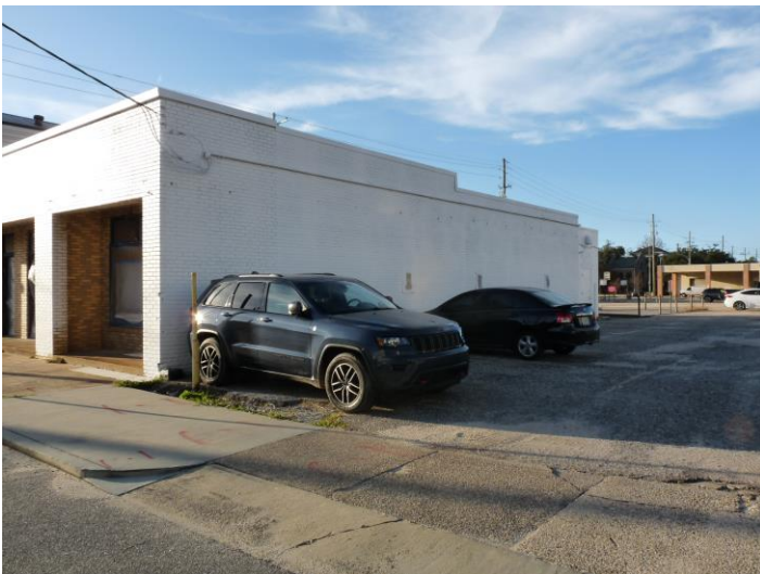
3. East elevation, looking northwest
