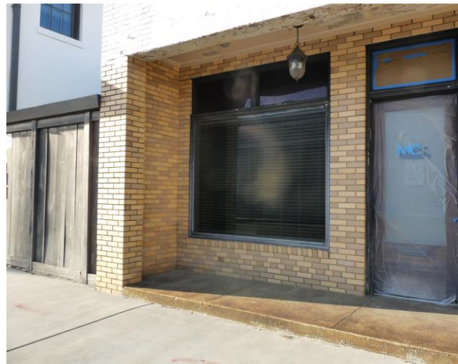
4. Detail of paint on façade
