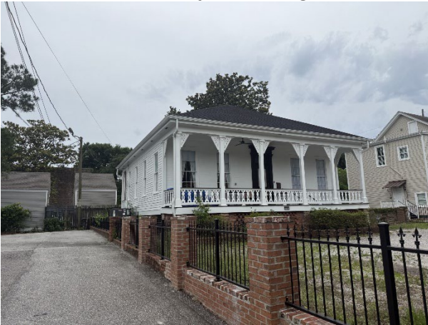
3. Northeast profile of existing structure.
