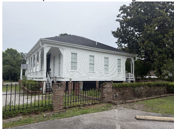
6. West side yard and west elevation of existing structure, looking E.
