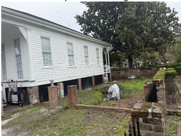
5. West side yard and west elevation of existing structure, looking S.
