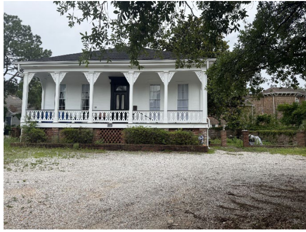
4. View of yard to the west of existing structure.
