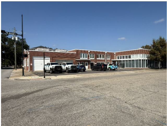
1. View of building looking NW
