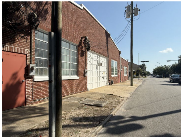
2. View of south elevation, looking NE
