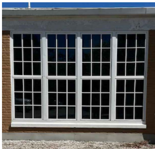
6. Existing windows that the proposed windows will replicate
