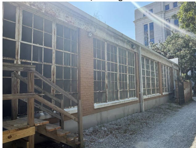
4. View of west elevation (windows to be replace looking SE)
