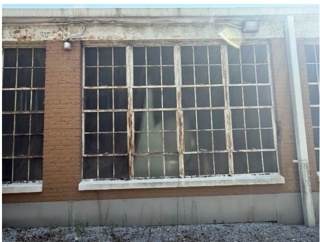
5. Detail of existing window condition
