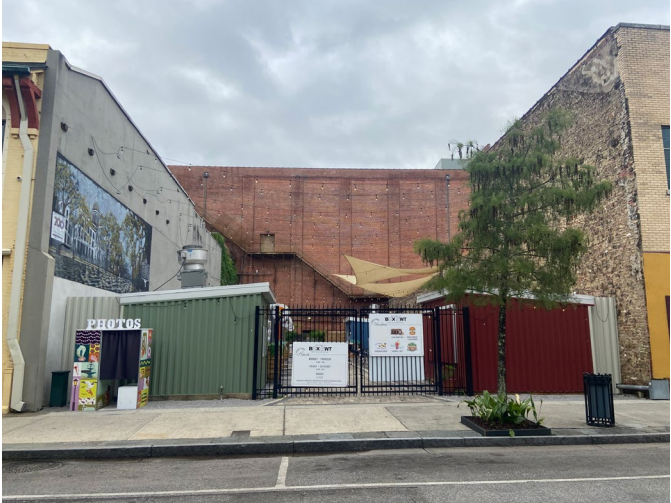
1. View of property, looking S
