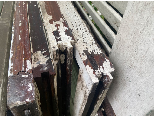
17. Detail of replacement one-over-one windows.
