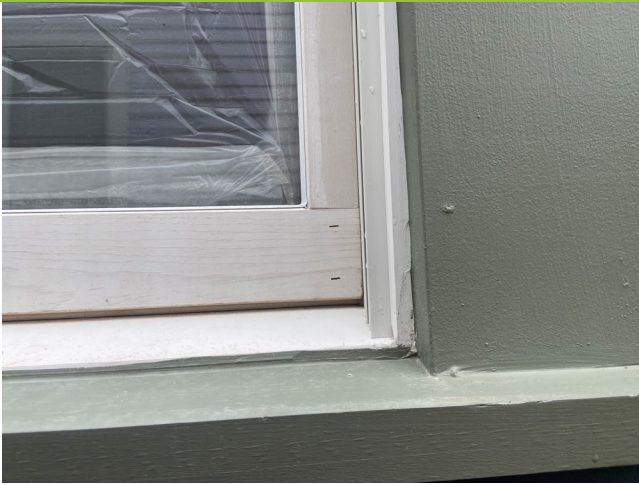
13. Detail of replacement one-over-one windows.
