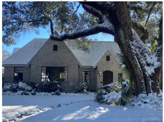
4. Gabled projections and stone cladding at 100 Levert Avenue, looking E
