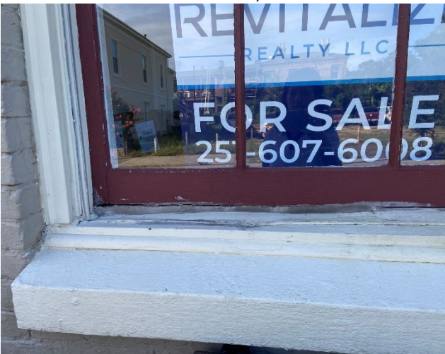
5. Detail of first-floor window, second from left
