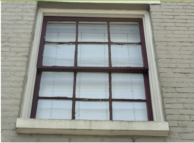
7. Second-floor window, first from left
