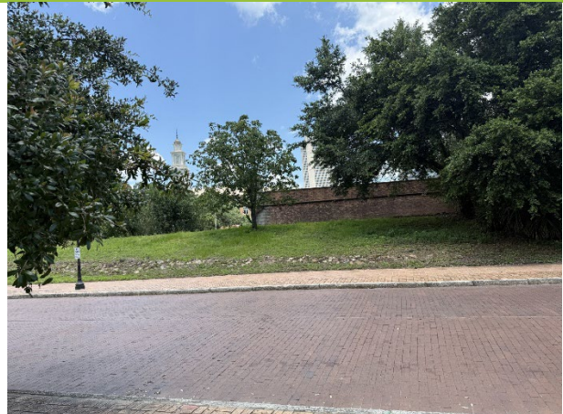
8. Masonry wall surrounding Fort Conde, looking N from Theatre Street.
