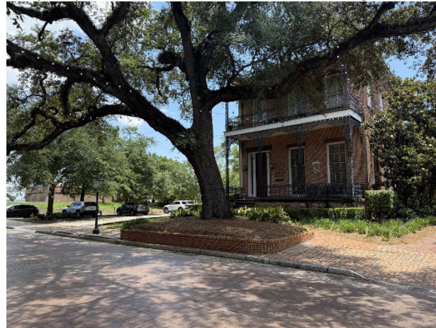
6. East façade of 163 St Emanuel Street and subject parcels, looking N.
