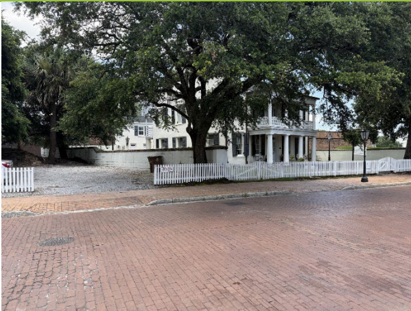
7. 104 Theatre Street and masonry wall, looking N.
