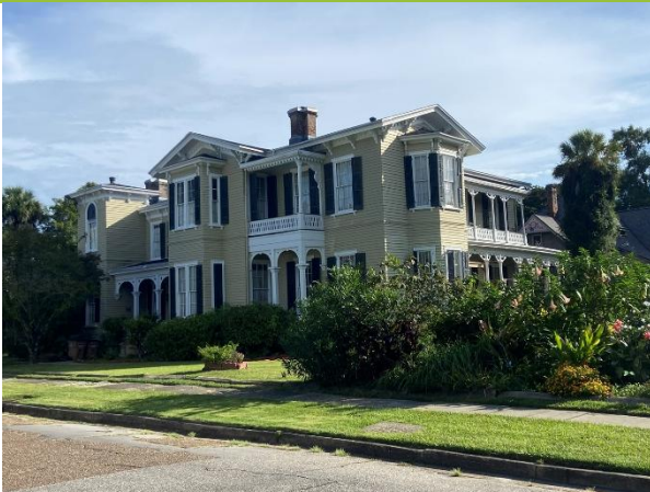
7. 1012 Palmetto Street at NE corner of Chatham and Palmetto, looking NE
