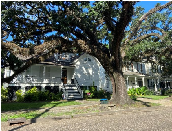
9. 210 George Street, looking W
