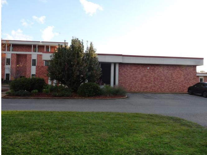
1. North elevation, looking south.
