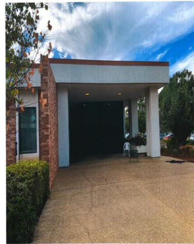
4. Existing covered patio area and screen enclosure, looking northwest.
