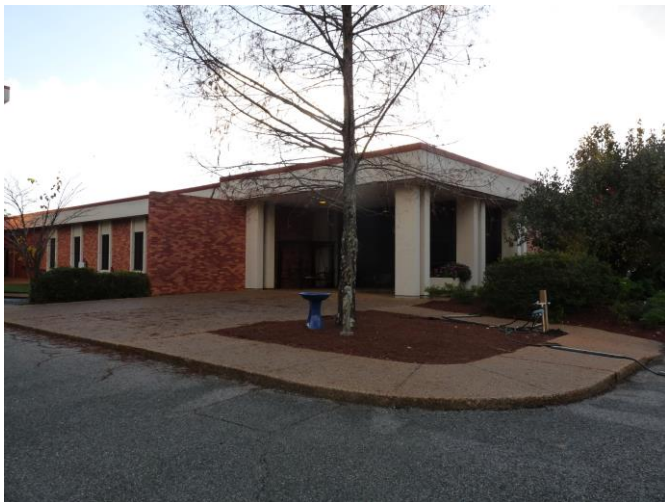
3. Existing covered patio area and proposed area for new screened patio. Looking southwest.
