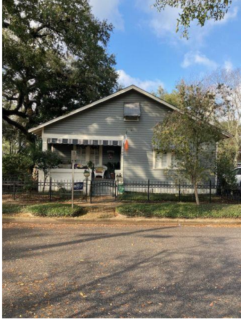
1. View of property's east façade, looking west
