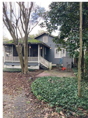
6. View of backyard, looking east.
