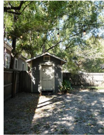
4. View of northwest corner of lot, looking north. (structure has been approved for demolition)
