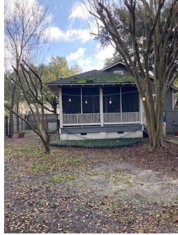
2. View of rear elevation, looking east.
