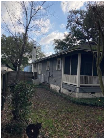
3. View of rear of structure, looking southeast.
