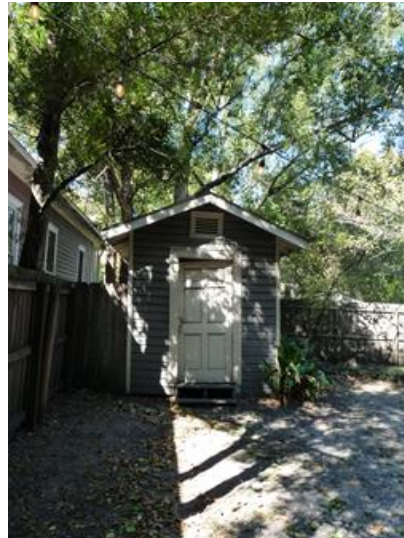
2. View of façade
