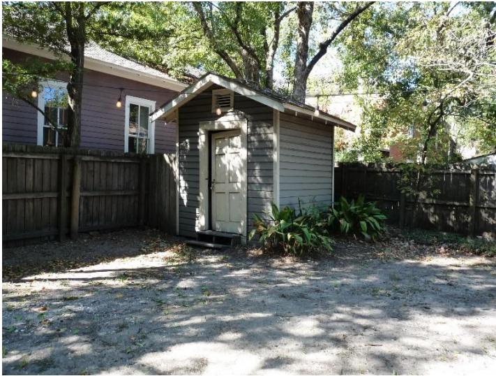
1. View of accessory structure looking north by northwest
