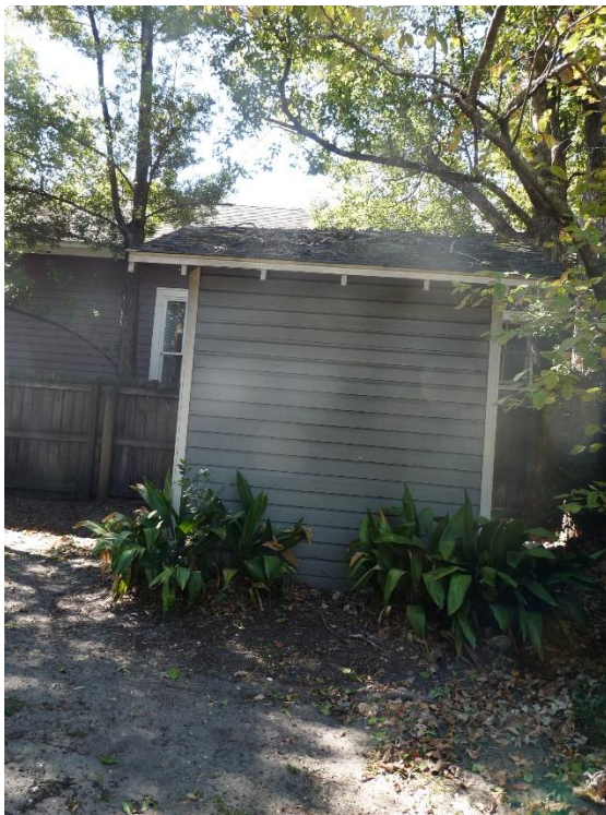
3. View of south elevation
