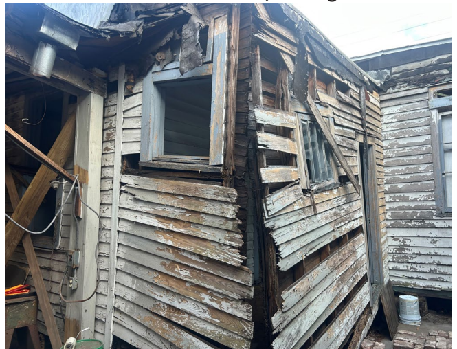
4. Detail of exposed exterior walls
