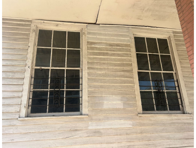
2. Detail of south elevation, looking N
