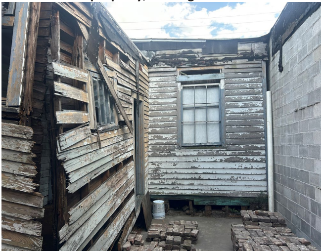
3. Details of exposed exterior walls
