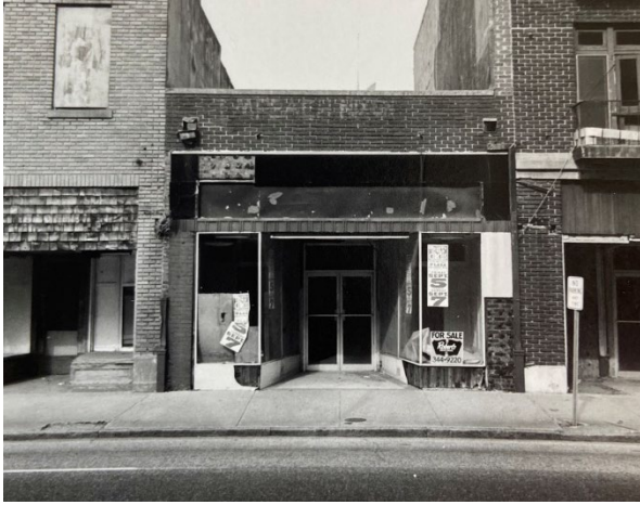
7. View of south facade in 1981, looking N
