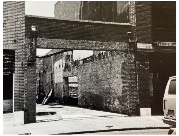
8. View of south facade in 1985, looking NE
