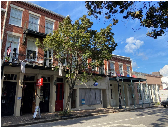
3. View of neighboring properties, looking NE
