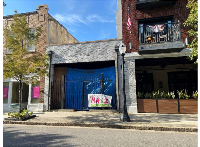
2. View of south facade, looking N
