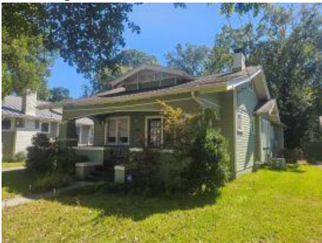
3. Façade and west elevation of 1565 Luling Street, looking SW
