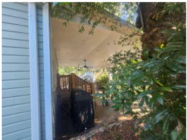
4. View of rear covered patio, looking W
