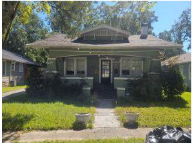
2. Façade of 1565 Luling Street, looking S
