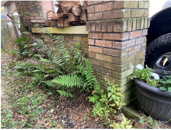
7. Mortar loss and vegetation growth at carport supports
