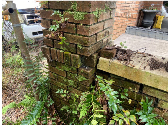
8. Mortar loss and displacement of carport supports
