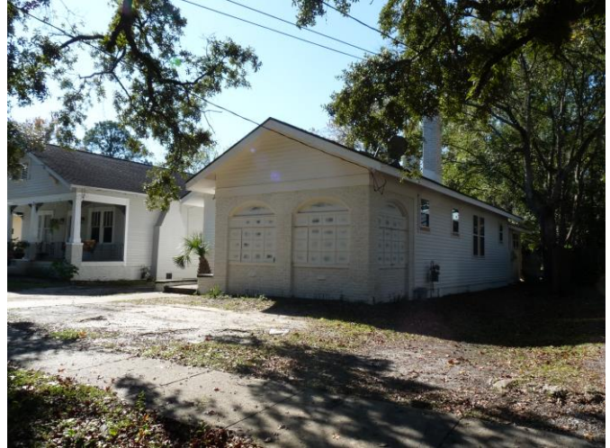
2. East elevation, looking southwest
