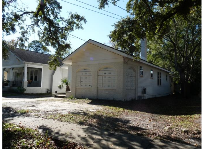
2. East elevation, looking southwest
