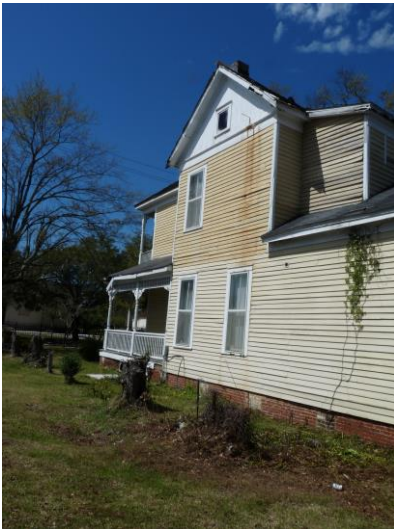
3. View of south elevation, looking northwest
