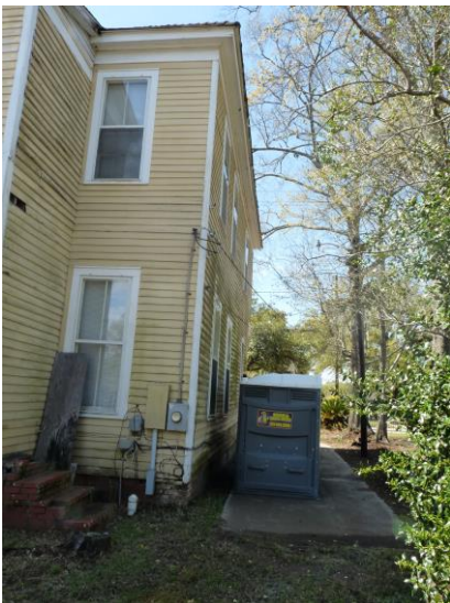
5. View of rear and north elevations, looking west
