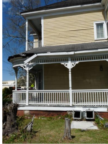
2. West end of south elevation
