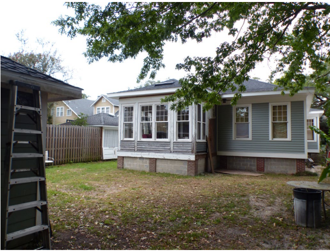
3. Rear (South) elevation of the main dwelling; northeast corner of teahouse at left
