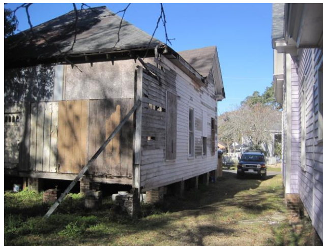
4. Rear and east elevation, looking northwest
