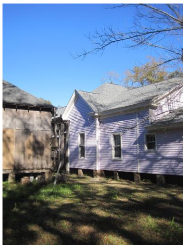
5. Rear elevation, looking northeast. Note partial wall to be removed.
