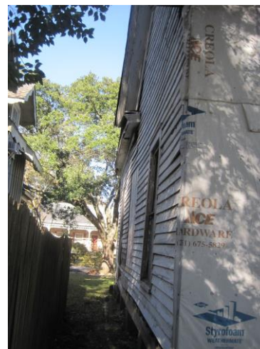
6. West elevation, looking north.
