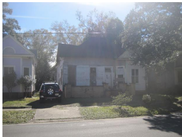
2. Façade, looking south
