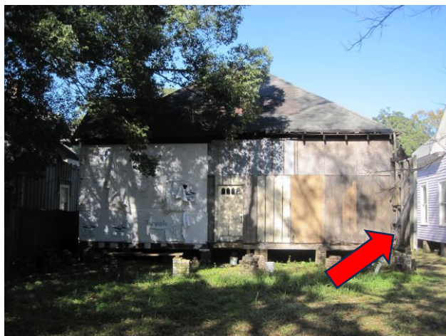
3. Rear (south) elevation. Partial wall to be removed can be seen on the east end.
