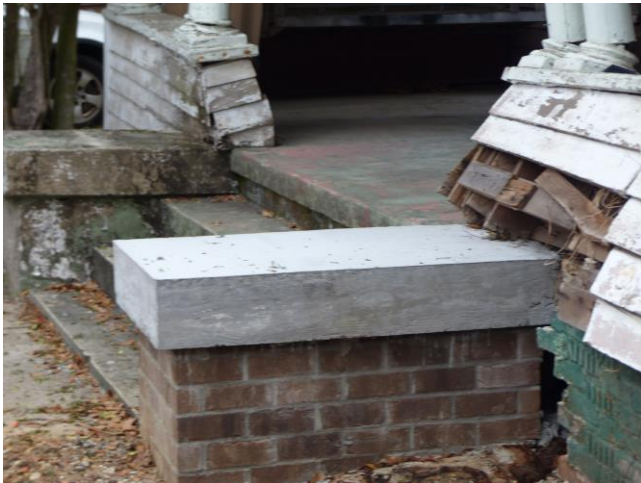
3. Detail: cheek walls, looking north
