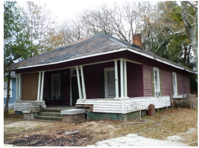
4. View of porch, looking northeast
