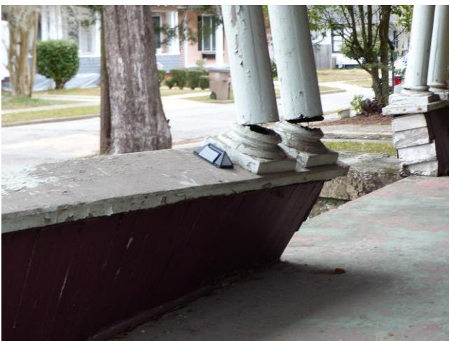
5. Detail: column bases, looking northwest
