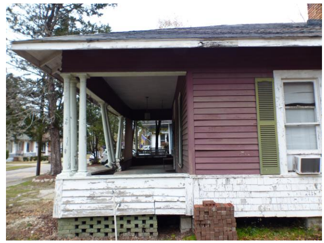
6. Side (south elevation), looking north
