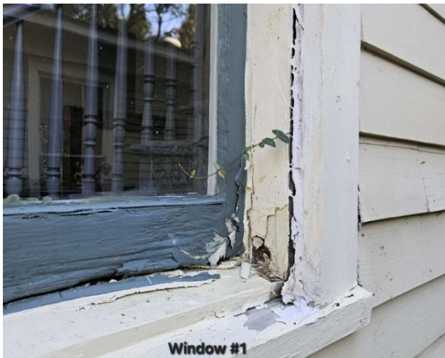
3. Applicant window survey: Window #1
