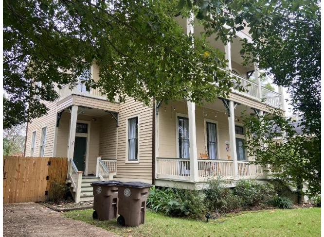
2. North and east elevations, looking SW
