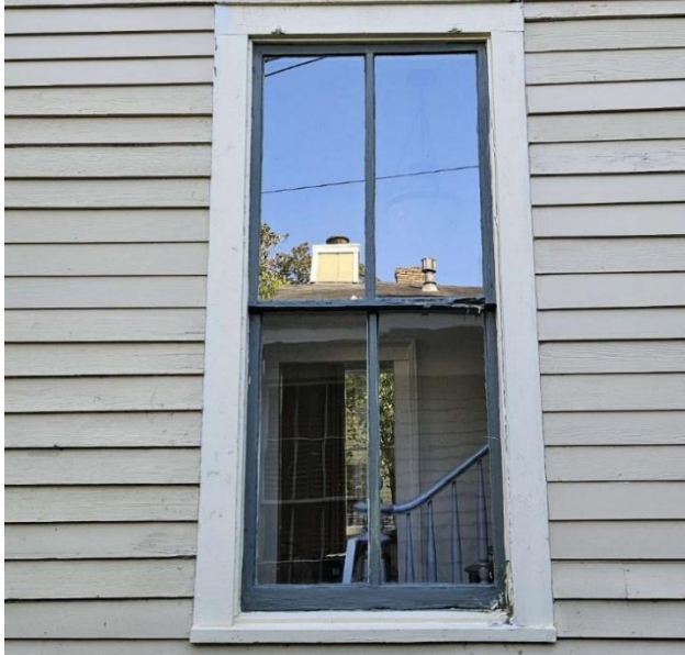
1. Applicant window survey: Window #1
