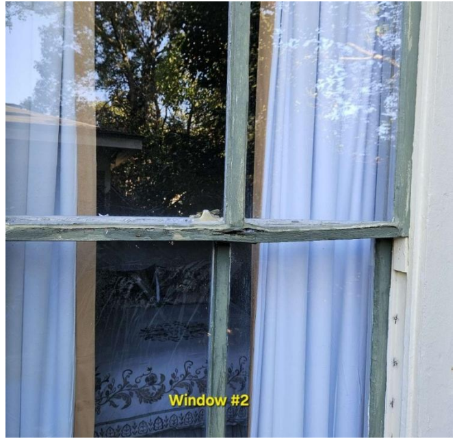
7. Applicant window survey: Window #2
