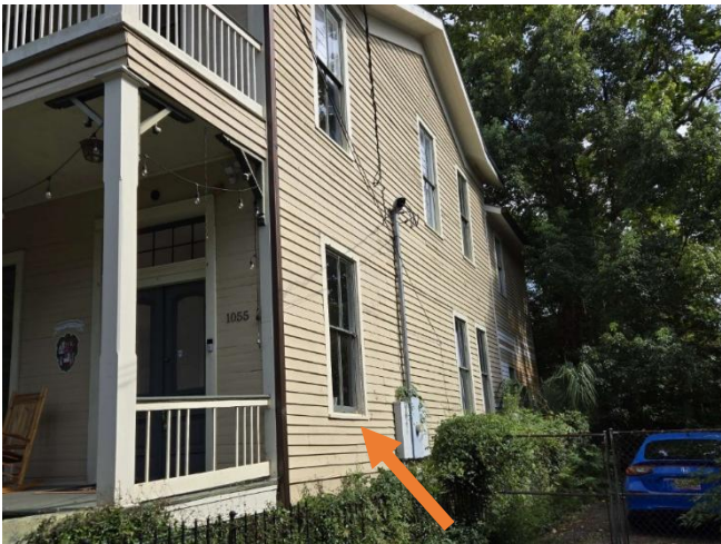
3. Location of Window #1 on west elevation, looking SE
