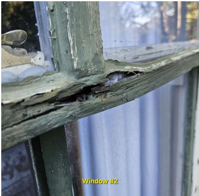
8. Applicant window survey: Window #2
