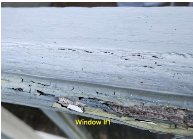
5. Applicant window survey: Window #1
