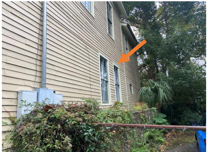
4. Location of Window #2 on west elevation, looking SE
