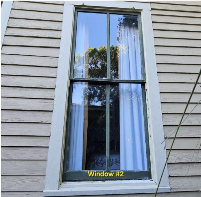
6. Applicant window survey: Window #2
