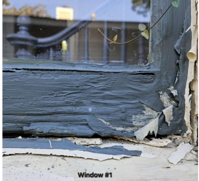
2. Applicant window survey: Window #1
