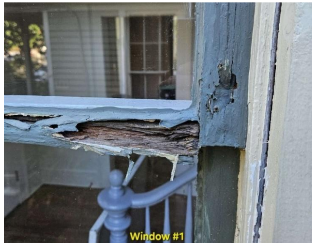
4. Applicant window survey: Window #1
