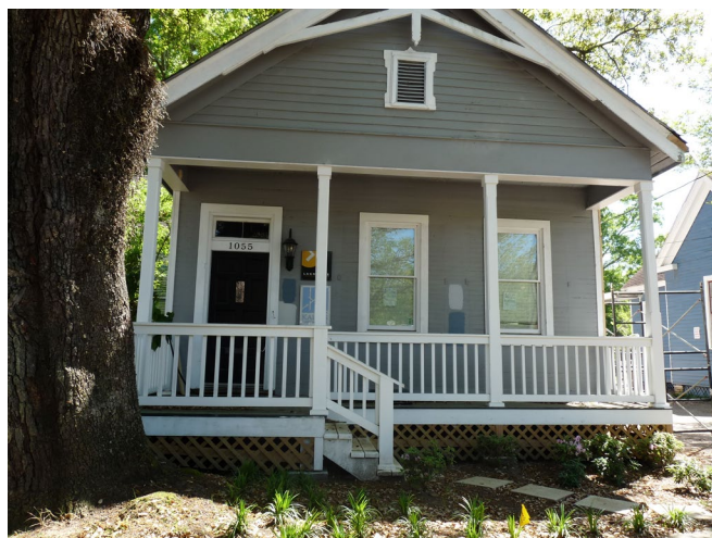
5. View of north façade, looking south.
