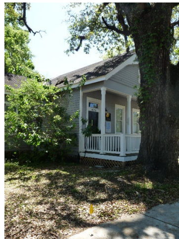
2. View of north façade and east wing, looking SW
