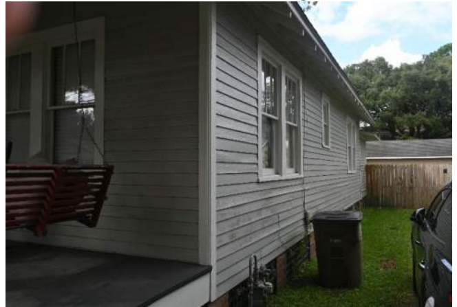
4. View of south elevation, looking NW
