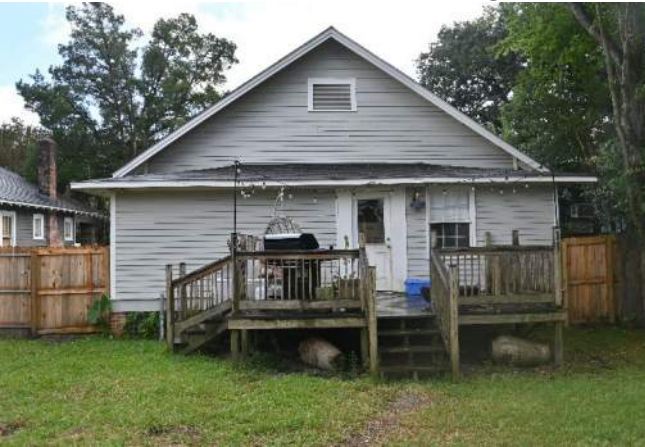
5. View of rear elevation, looking S
