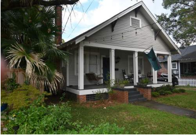
1. View of south structure, looking NE
