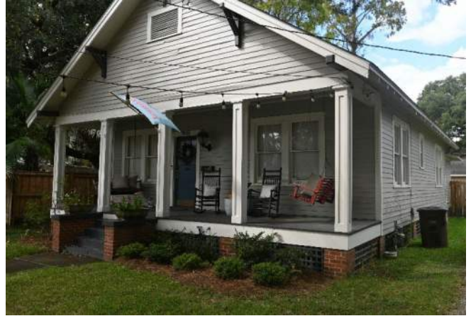
2. View of structure, looking NW
