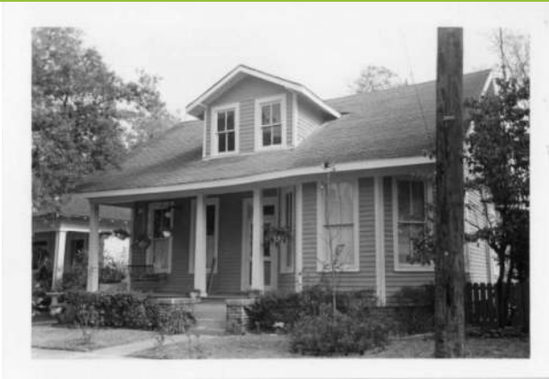
7. West façade, looking NE (MHDC survey photo, 1988)
