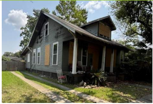
2. West façade and north elevation, looking SE
