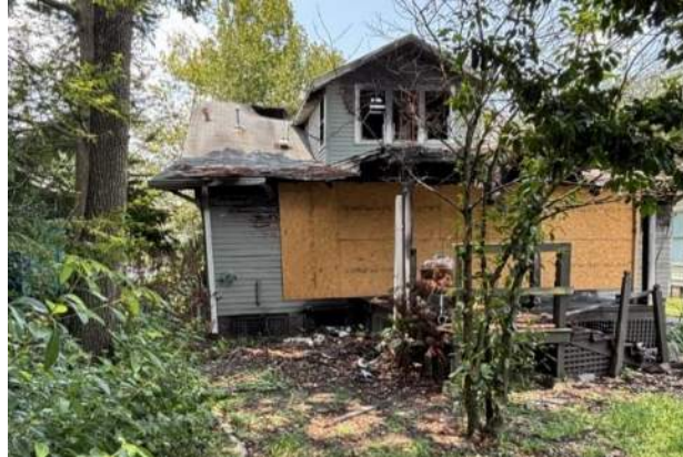
4. East (rear) elevation, looking W
