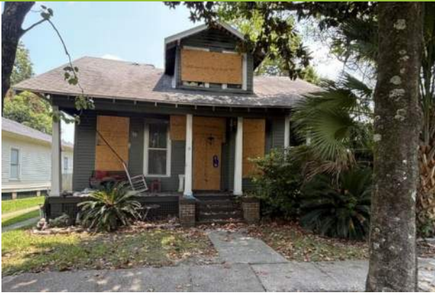
1. West façade, looking E
