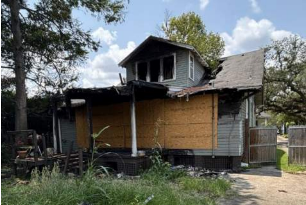
3. East (rear) elevation, looking W
