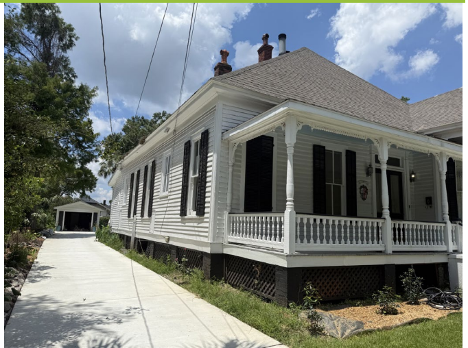
2. View of elevation, looking NW
