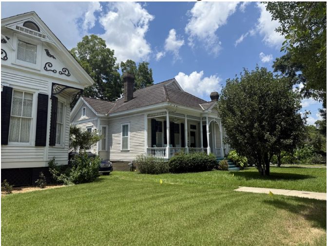
5. View of neighboring property to the with similar roof form. Looking NW
