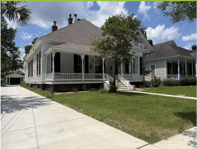
1. View of property, looking NW
