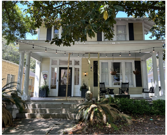
2. Location of removed columns, looking E
