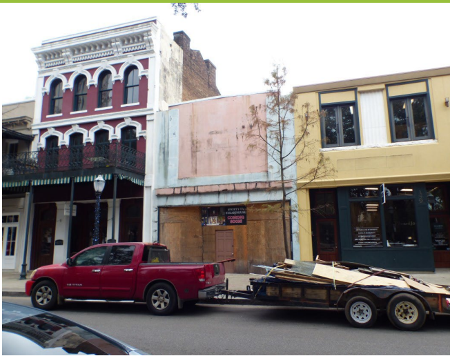
1. View of 157 Dauphin, looking south
