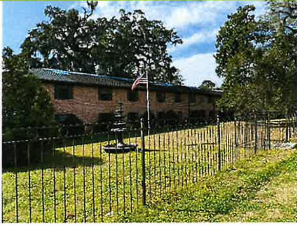
1. North façade of 1621 Springhill Avenue and existing fountain.
